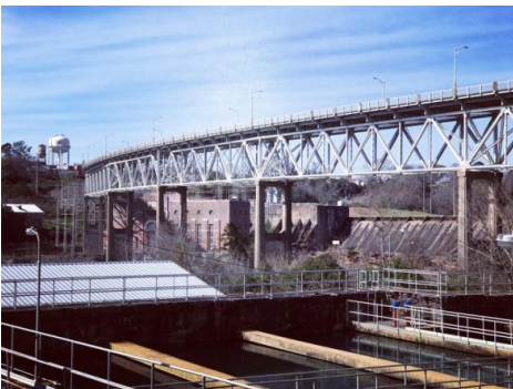
The City water filtration plant is located on the bank of the Tallapoosa River.
