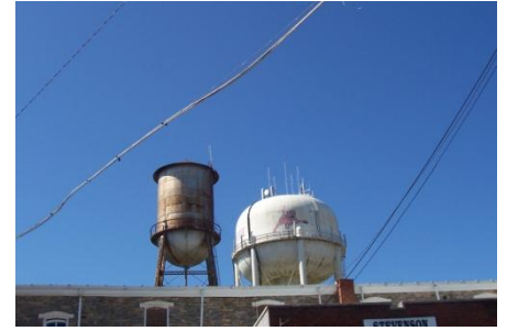
Two of Tallassee's water towers are located in the downtown area.
