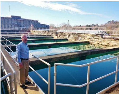
Steve Oswalt, former supervisor of the water filtration plant, standing next to the facility's treatment pools.
