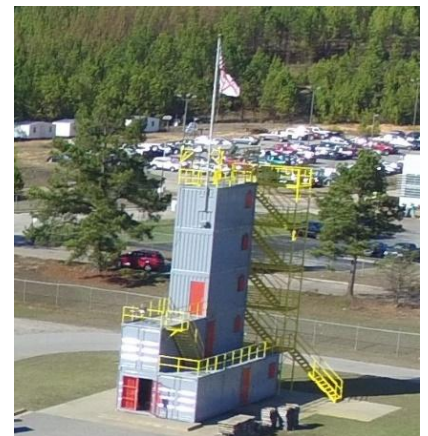
Fire Stations No.1, No. 2, No.3 and Tallassee's Fire Training Facility.
