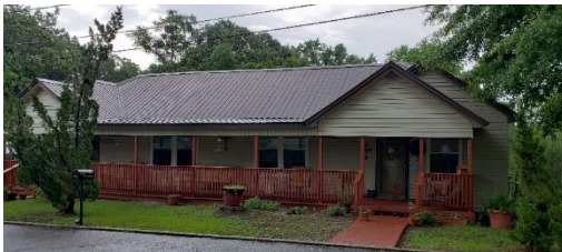
A renovated duplex residence in one of Tallassee's mill neighborhoods.
